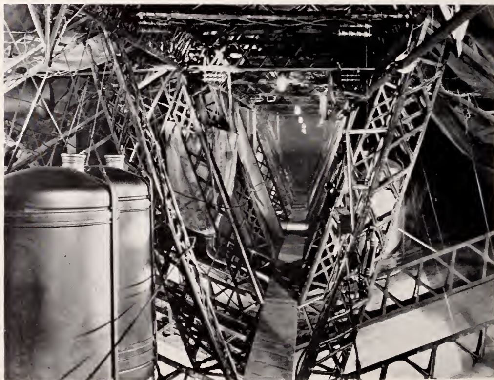
A view down the "Catwalk" of the "Los Angeles"
